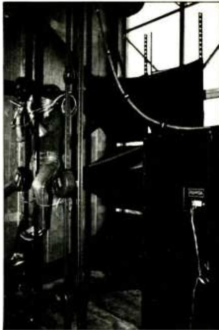
**Figure 1: dB Sound crew installing Panasonic WU-566/2 driver on WU-5948 long throw horn for L.A. Coliseum main speaker cluster.**
