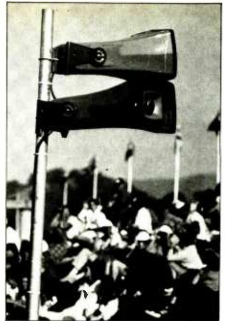
Figure 9: Panasonic long-throw horns were used at Lake Casitas to cover the 10,000-capacity spectator area for canoeing and events.
