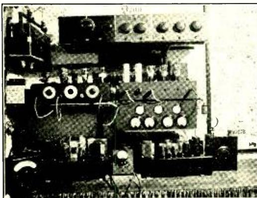
Two transmitters are used at ZUIT. One is used on 20 and 40 meters; the other is for 10. A 66 foot zepp. is used on 20 and 40 meters. A 67 foot single-wire-fed antenna is used on 40, 20, and 10 meters.
