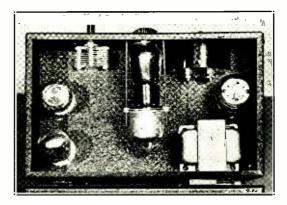
Looking Down into the Monitor, Showing Method of Mounting the "Magic Eye" Tube.
