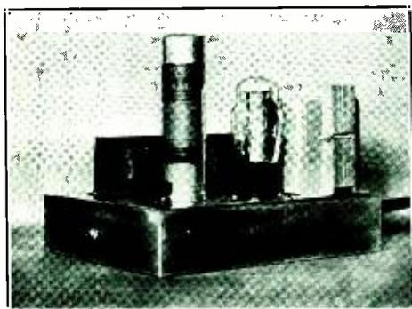
The Power Supply and Speaker Coupling Unit
