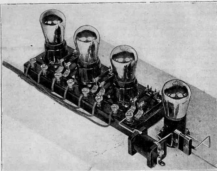
Method of Installing R.F. Choke Ahead of Resistance Coupled Amplifier.
