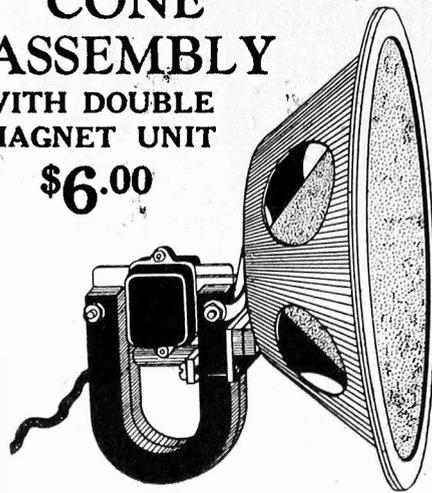
An excellent magnetic type speaker for installation in any cabinet. The unit is a double-magnet Paratone, with two magnet coils, for utmost sensitivity. Each horseshoe magnet is 3/4" thick. The magnet coils are forever protected against dust and other foreign, injurious substances, by special bakelite housings. The pin is reverse drive. The cone frame is metal. The 9" cone is specially treated buckram.
