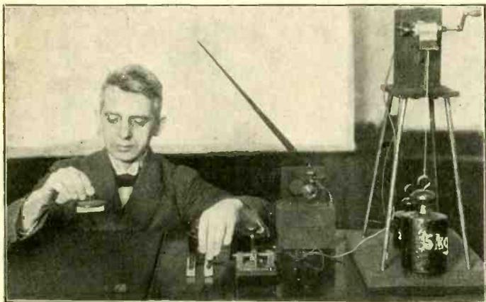
Fig. 1. Fundamental test of a new electrical phenomenon showing a metal plate clinging to a stone slab during the passage of a minute electric current.
