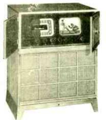
AM-FM CONSOLE in rich mahogany. AC, 8 tubes plus rectifier. Permeability tuning with 5 push buttons for AM band. Inverse feedback, RF stage for both bands. Two built-in antennae. Three-position tone control. Picture clear Strobo-Sonic Tone!
