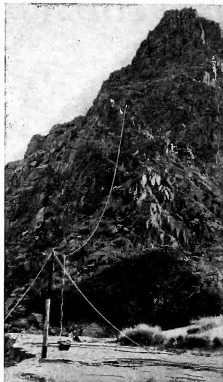
Antenna installed in Grand Canyon of Colorado River for receiving radio messages for the Geological Survey, U. S. Department of Interior.
