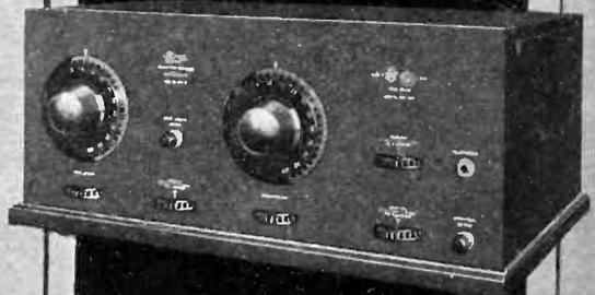
Type CR-14 — A 3-tube dry cell Regenerative Receiver . . . . \$110.00
