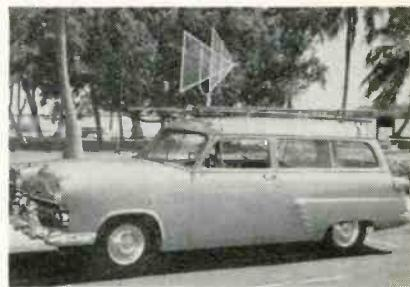
Convinced that TV antennas could best be sold by actual field demonstrations, American Screen Products Co. of Miami outfitted this mobile unit with their Unicorn antenna, a telescoping mast, TV receiver and field strength meter, and sent it out to roam the Florida Gold Coast. The result—discovery of brand new TV fringe areas, and valuable data for local servicemen and TV engineers.
