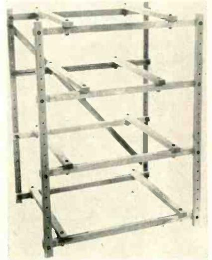
rack, of wood construction and secured by thumbscrews and bolts, can be adapted to accommodate units requiring different amounts of head room and shelf space. Retail for \$9.90. River Edge Industries, River Edge, N. J.—TECHNICIAN.
