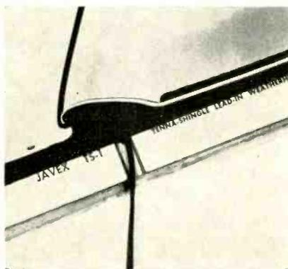
in. The Tenna-Shingle is transparent, and takes on the color of the surface to which it is attached. It accommodates standard 300-ohm twin-lead line. Javex, Redlands, Calif.—TECHNICIAN.
