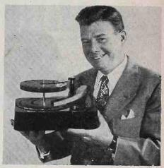
10" and 12" records, all automatically. Cartridge uses a replaceable sapphire tipped needle. List price on the model 104 is \$16.95. Columbia Records, Inc., 1473 Barnum Ave., Bridgeport, Conn.-RADIO & TELEVISION RETAILING.
