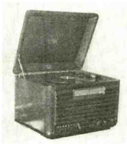
sole quality) can be easily adjusted for desired amplification. Push-button and manual tuning; life-like fidelity. 5 watts output. Phonograph mounted on floating springs and thoroughly insulated. Plays 10" or 12" records with lid closed. Built-in loop antenna. Tunes to 535-1620 kc. Measures 18" x 14 1/2" x 12". Music Master Radio Corp., 750 Main St., Hartford, Conn.—RADIO & Television RETAILING
