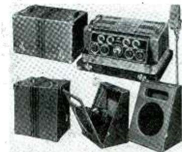
**SOUND SYSTEM**—High powered portable sound system Model C-483 rated at 40 watts output. Has 4 microphone inputs with gain of 128 db.
