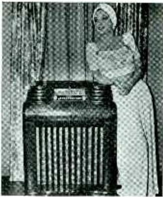
**LOWBOY CONSOLE**—Push-button tuning; slide rule dial; matched walnut, hand-rubbed cabinet; 9-tube superhet; foreign and police band reception; has a dual directional loop antenna that eliminates the need for outside or inside aerials and trailing wires.
