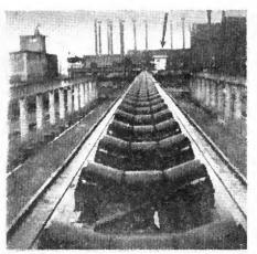
The beets then go onto this 1200-ft. conveyor (belt not in place in photo), travel to the small "tare" house in the distance, 18-feet above ground, where 15 lb. samples of every load have dirt wire-brushed off, tops removed
