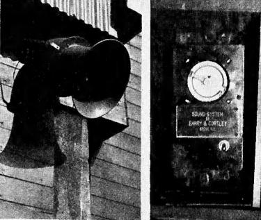
**CONSTRUCTION** Final link of New York's Tri-borough bridge is raised into position 135 feet above East River. War Department allows 6-hour maximum for job, *Davie Electric Company* equips foreman (arrow) with microphone, installs six speakers (cireled), runs 100-watt amplifier on a.c. cabled from shore. Co-ordinating directions audible to hoist operators (tower tops), steelmen and fireboats pumping water into float on which span was towed into position. Time: 5½ hours
