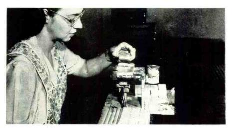
Fig. 4. Silk-screen printing. Paint is farced through the open mesh of the screen. After the screen is removed, the surface of the base plate is found to be printed with an exact, sharp-edged, uniformly-thick design of the required conductor circuit. A second stencil can then be used to print the resistors in their proper location.
