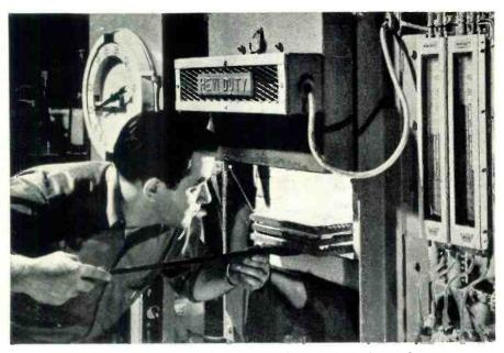
Fig. 6. A high temperature oven is used for firing a group of printed circuits.
