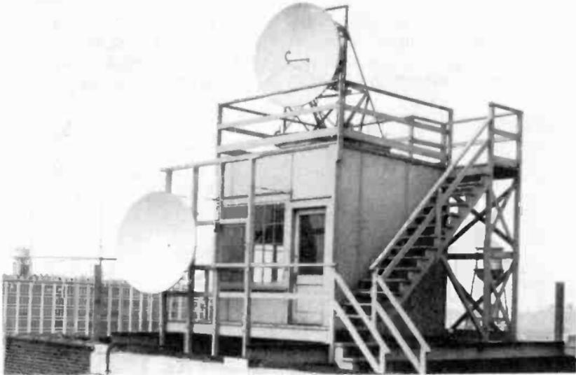
Figure 104. Permanent installation of microwave relay antenna.
