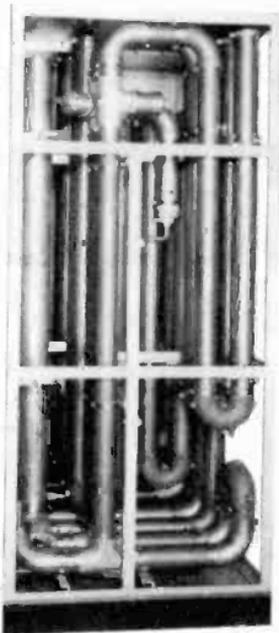
Figure 110. Vestigial sideband filter. (courtesy RCA)
