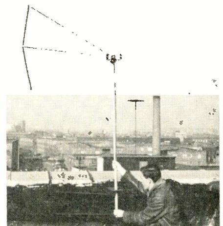
Wooden masts, made from broomsticks, made perfectly good supports for the simpler types of antennas in many cases. Shortages of steel masts have made these installation feasible in many TV localities.
