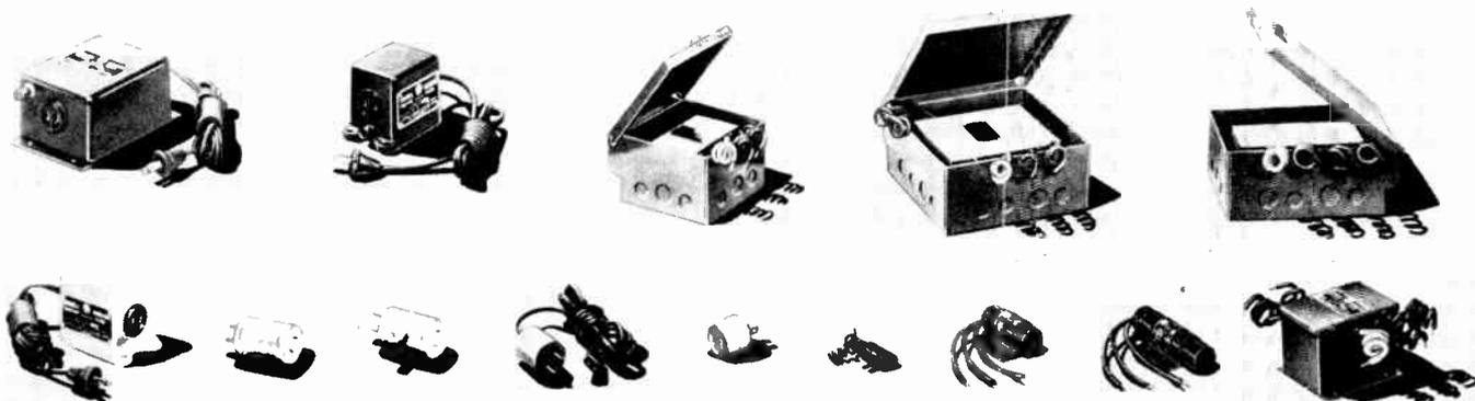
A GROUP OF INTERFERENCE FILTERS MANUFACTURED BY CORNELL-DUBILIER. LIGHT AND HEAVY DUTY UNITS ARE SHOWN WITH MOUNTINGS SUITABLE FOR THE USE TO WHICH THEY ARE TO BE PUT.
