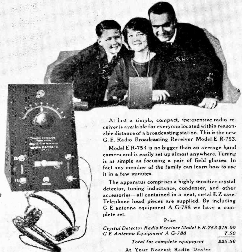
Fig. 2 One of the few crystal sets which were built commercially for home use is described in this advertisement, which appeared in 1922.
