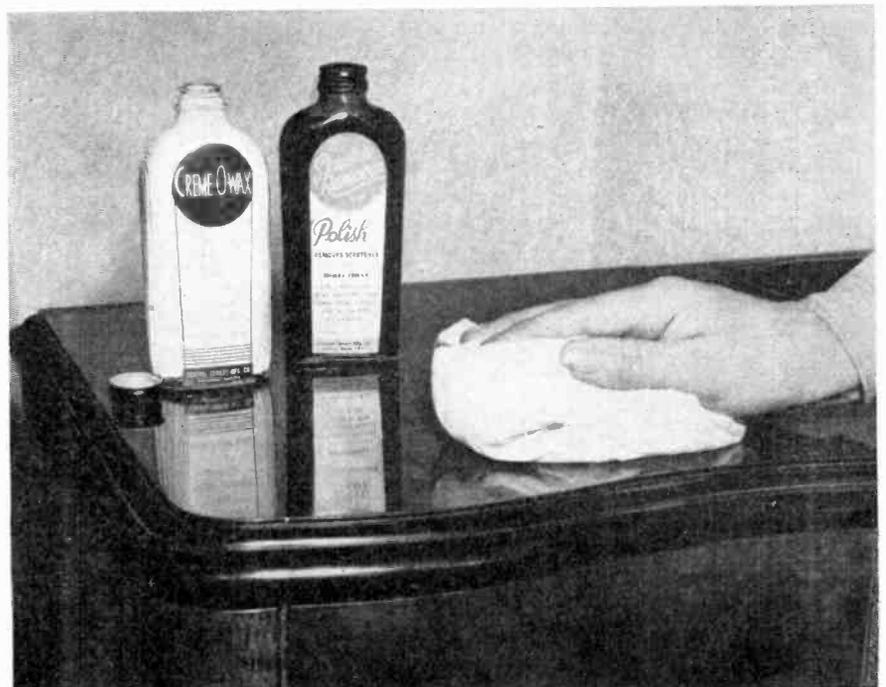
Fig. 2 Applying scratch remover and polish with a soft cloth.
