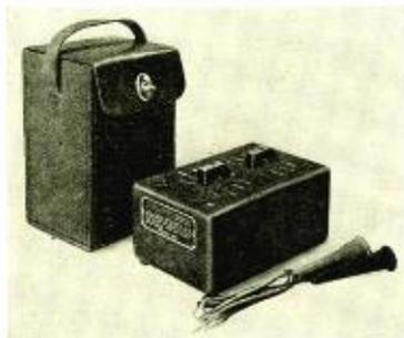
to tell the correct condenser capacity for a circuit, enabling a wide variety of capacities to be cut in until the right one is obtained. Besides giving the correct capacities for those that have actually broken down, the indicator makes it possible to check the efficiency of all the condensers in the set, it is stated.
