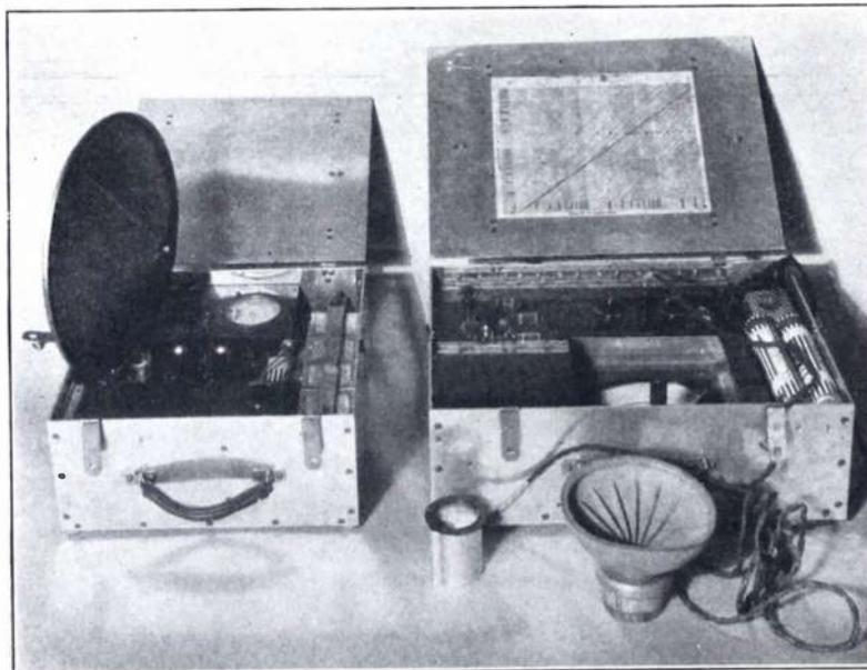
The complete Acoustimeter equipment. The pick-up and the indicating meter can be seen in front of the right hand case.
