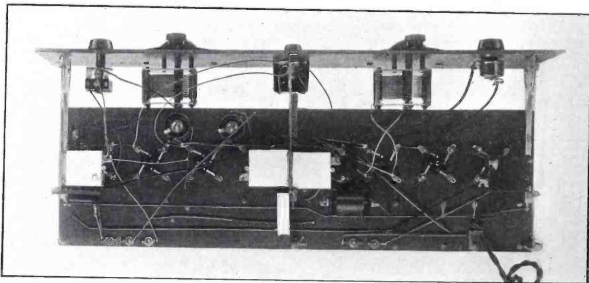
Bottom view of the new Victoreen. The potentiometers controlling the second and third intermediate tubes are mounted on the sub-panel, as shown. Flexible connections are made between the front panel apparatus and the sub-panel units and, since the mounting brackets are adjustable, a sloping front cabinet can be used, if desired.
