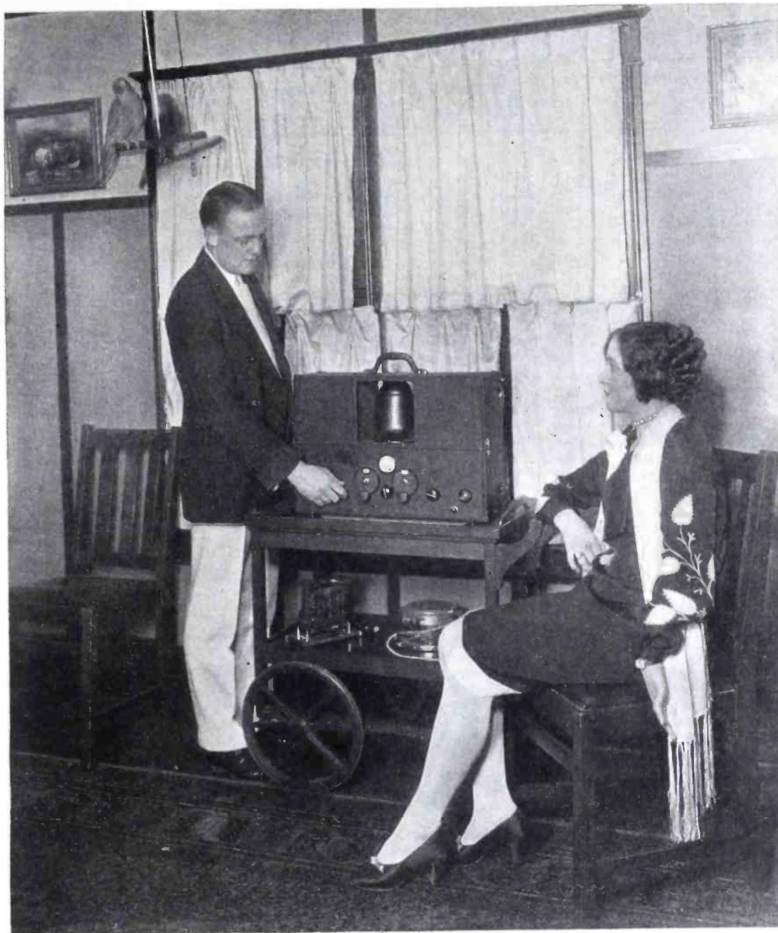
Complete set up of the Portable Super. The design of this receiver has been so worked out that it is adaptable to practically any installation requirements. Sufficient space is available in the cabinet for dry batteries, so that the outfit can be moved easily.
