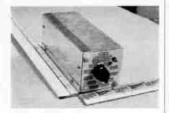
to find a frequency. Simple to install, the "Selecto-Tuner" operates on all frequencies between 118 and 130 mc. It is 2%" square by 6" long, and weighs seven ounces.
