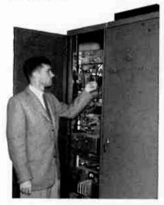
New stylized racks with doors feature modern functionalized design and open back for ease of servicing. Open cabinet shows complete Microwave Terminal. Closed rack shows stand-by equipment.
