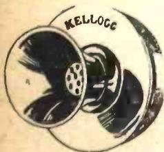
Regular telephone transmitters taken from a large telephone supply company's overstock. Work perfectly on 2 dry cells. Can be used on P.A. systems, call systems, intercommunications sets, short-line telephone circuits, house-to-house or farm-to-farm 'phone lines, also to talk through your own radio or as concealed dictaphone pick-up. Useful replacements on battery-operated rural telephone lines.
