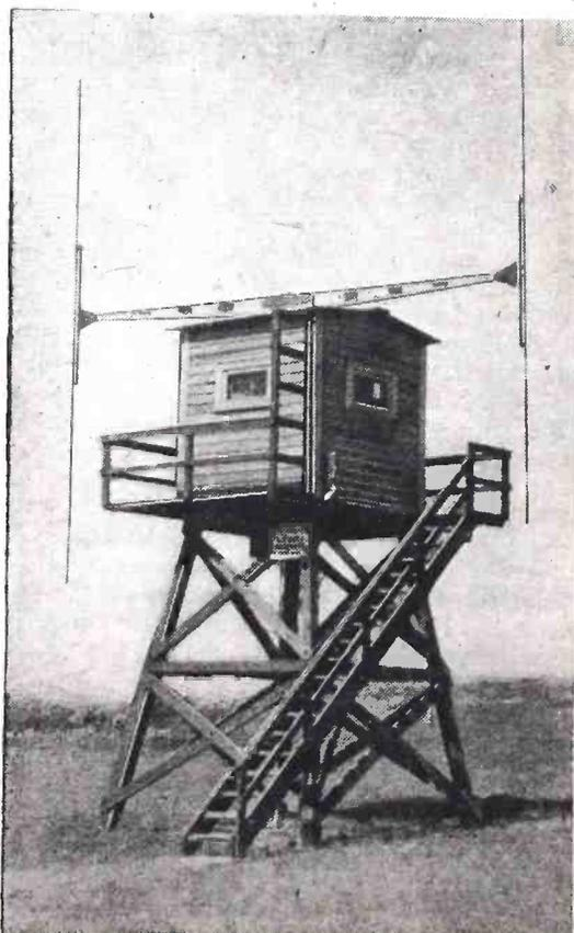
The Adcock apparatus, for long-distance work.
