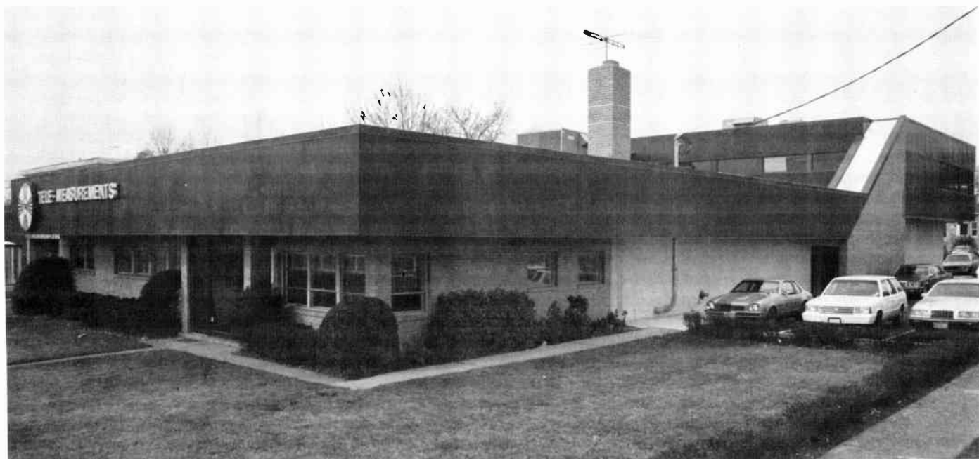
Tele-Measurements, Inc., 145 Main Avenue, Clifton, New Jersey.
