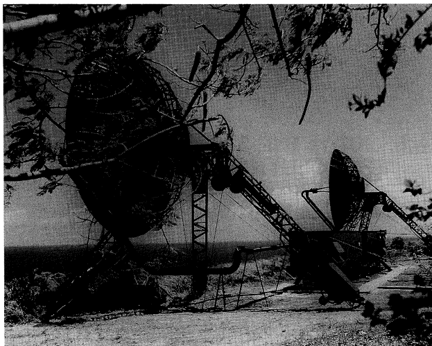
Figure 11. AN/MRC-98 Transportable Terminal, operating at 755 - 985 MHz. with 30 foot transportable antennas.
