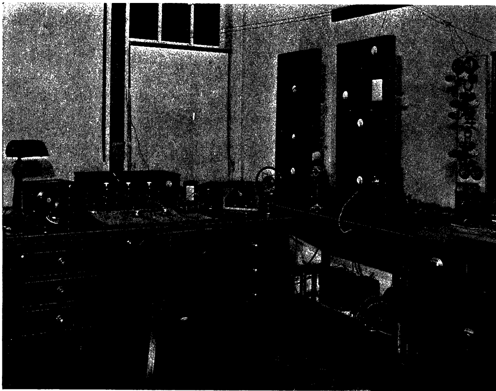
Station "W2GEC". G. E. Burghard, 520 East 86th St., N. Y. C., 1934. Left to right: Frequency meter, single signal superhet, 5 meter super-regenerative receivers, Modulator panel, C. W. transmitting panel, 20 to 180 meters, and 5 meter M.O.P.A. transmitter.
