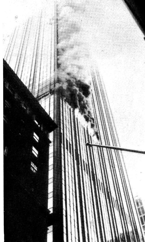
Fig. 1. A typical hi-rise fire.
