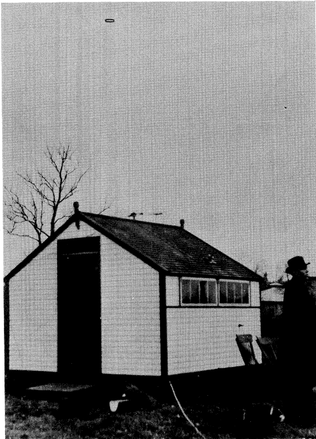
Armstrong at right, supervising construction.
