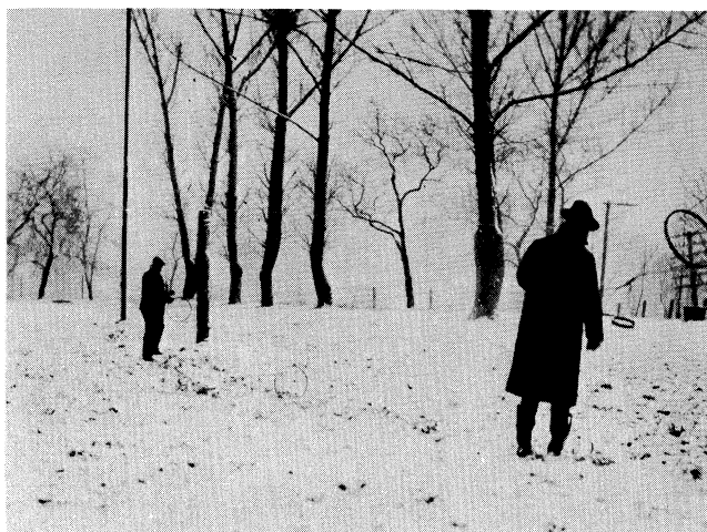
Getting ready to hoist the cage antenna.
