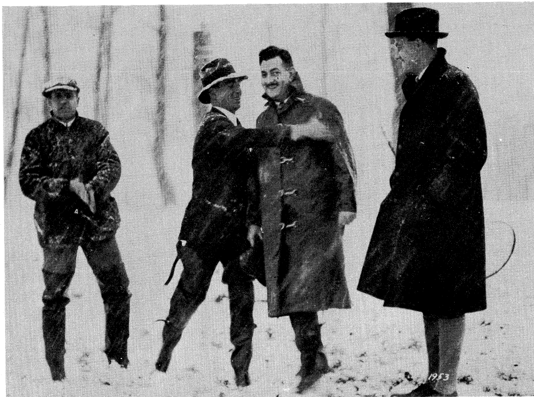
Time out during the building of the counterpoise to warm up. Left to right—Burghard, Inmann, Grinan, Alva B. See.
