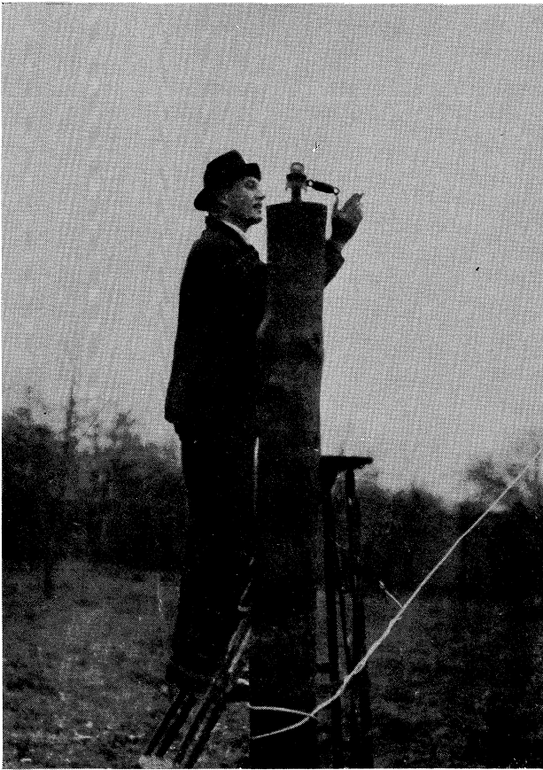
Amy inspecting the counterpoise during construction.
