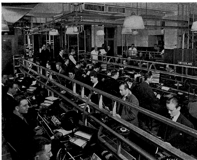
Fig. 1—General View of Telephone Room.
