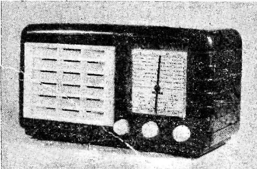
This Ultra Table Model has a plastic cabinet and speaker joint. It is a two-waveband model.
