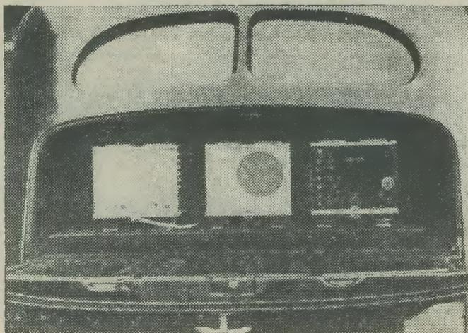
The complete equipment in the boot of a patrol car. Left to right—receiver, power unit and transmitter.
