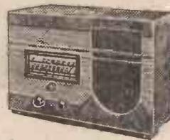
149. All-Wave Battery Receiver, 3 valves. 18-50, 195-560, 785-2000 metres. **9 1/2 GNS.**
