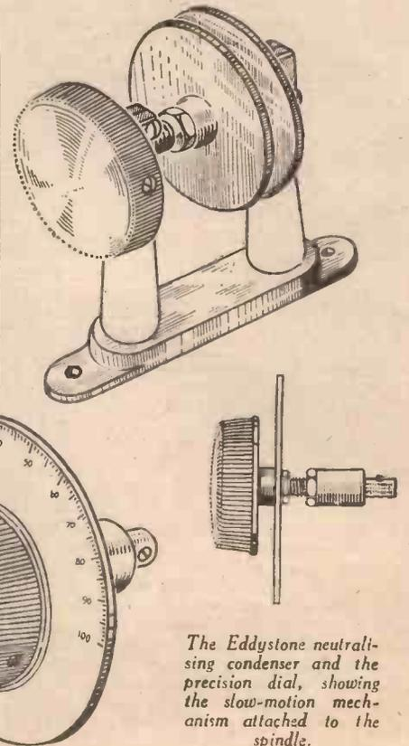
The Eddystone neutralising condenser and the precision dial, showing the slow-motion mechanism attached to the spindle.
