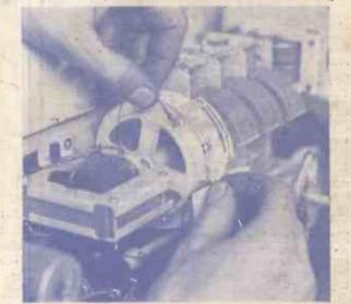
Another splendid illustration showing the fitting of a New Cord to the Drum of the Marconiphone 42
