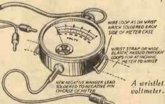
the common negative to the pin at the base of the meter, an extra lead can be soldered to this pin, as shown in the sketch, to facilitate use when the meter is attached to the wrist.
