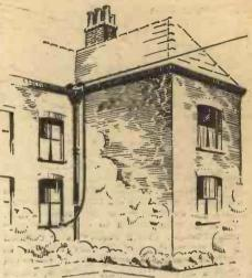
1,-Aerial and lead-in running close to gutter and rainpipe.
