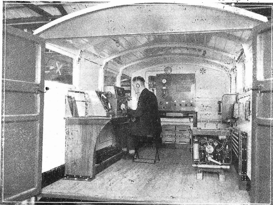
One of the motor "trailers" fitted with Marconi transmitting and directional receiving apparatus as installed for the British Air Ministry at the Hull, Belfast, and Portsmouth aerodromes. In this photograph the apparatus is shown undergoing tests; under service conditions, the receiving equipment, and switchboard for controlling the transmitter remotely, are usually removed from the lorry or trailer together with the operating table shown on the left of the photograph.
