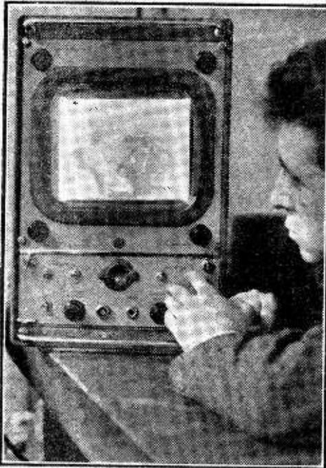
A closed-circuit TV system is now in use in a store in France to detect shoplifters. A hidden detective scans the counters by means of a TV camera mounted near the ceiling.
