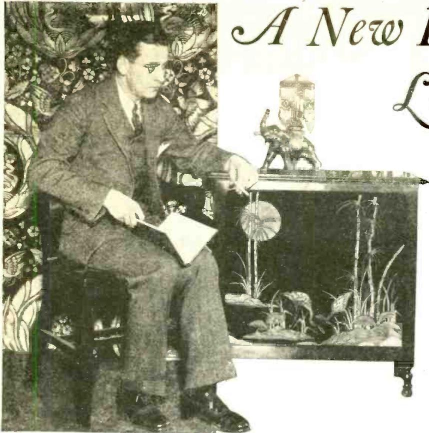
The familiar cone and horn types of loudspeakers have, at last, a serious rival in this new type of reproducer that operates on the principle of "balanced tension" between two tightly stretched skins. So extraordinary have been the results with the Air-Chrome loudspeaker, which incorporates this principle, that great popularity is predicted for it by radio experts who have heard it
