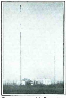
The antenna system of the Prague station was described as an Alexanderson type with three leads.
