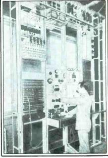
This shows the Dixon transmitting station's line terminal equipment. The room was totally shielded in copper to keep out stray RF.
