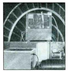
The Western Electric two-way communications equipment installed in Amelia Earhart's plane was assigned the callsign KHABQ.
