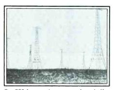
Six 280-foot steel towers at Japan's Komuro receiving station supported an antenna array that assured optimum reception of signals from America.
