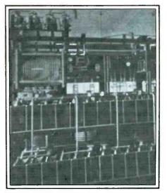
"Radio Journal," using the callsign OKP, in Prague, used this Western Electric 5-kW transmitter during the late 1920's.
