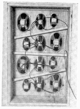
Speakers of different sizes permit unequal spacing between speakers and staggered resonances, alleviating two of worst faults of multiple speaker systems. But problem of restricted fundamental bass response and high-frequency dispersion remains.
