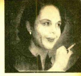
TELEVISED by the glow of a single cigarette, the picture above demonstrates the light sensitivity of a closed-circuit television that is said to amplify light up to 40,000 times.
