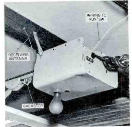
**Perma-Power Operator Installation**
