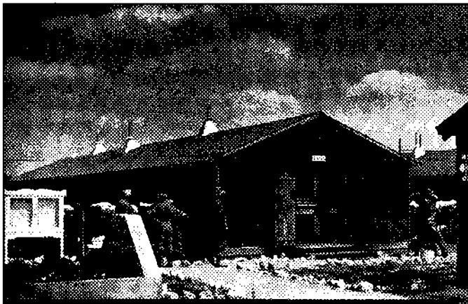
CAMP CROWDER: Housing for 66th Signal Battalion was called "Old Shanty Town" because of its tar paper barracks, heated in winter by small cast iron stoves.
