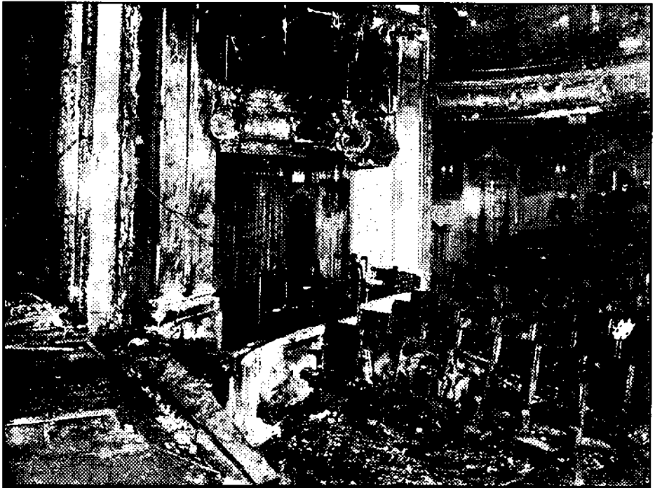
Interior view of the Iroquois showing the stage area where fire ignited draperies and spread quickly to combustible scenery props.
