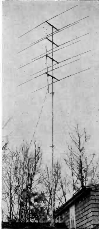
Fig. 3. Strong and light magnesium antenna mast, for heights of less than forty feet.
