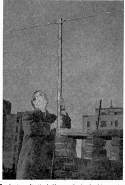
For best results the half-wave dipole should extend at least 10' above the roof of a building. Fig. I shows how the antenna is connected to a typical receiver terminal strip. You can use other types of low-loss feeders in place of the coaxial cable. If you do, connect one wire of the pair to each of the dipoles, and one to each of the first two terminal posts. This directional antenna favors signals coming from the directions shown by the blocked arrows.
