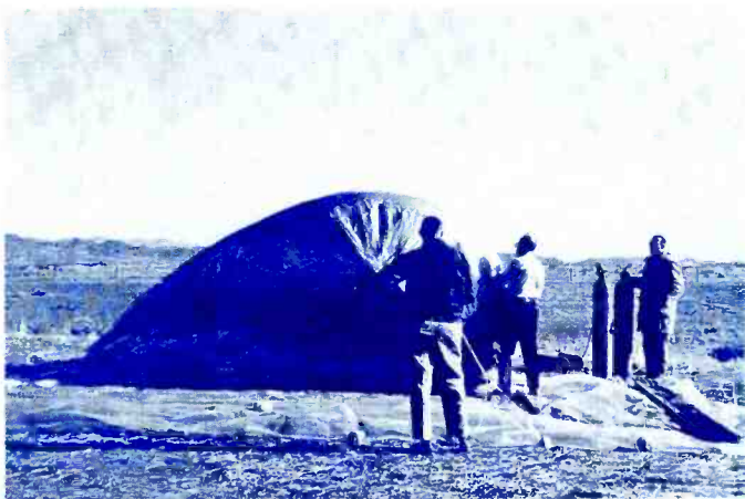
C. INFLATING THE KITE WITH HYDROGEN.
