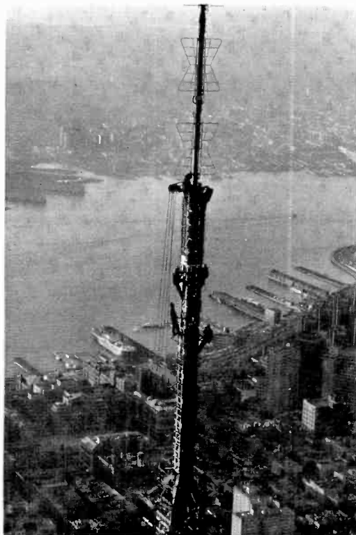
Fig. 11 Work in Progress on WPIX Antenna
