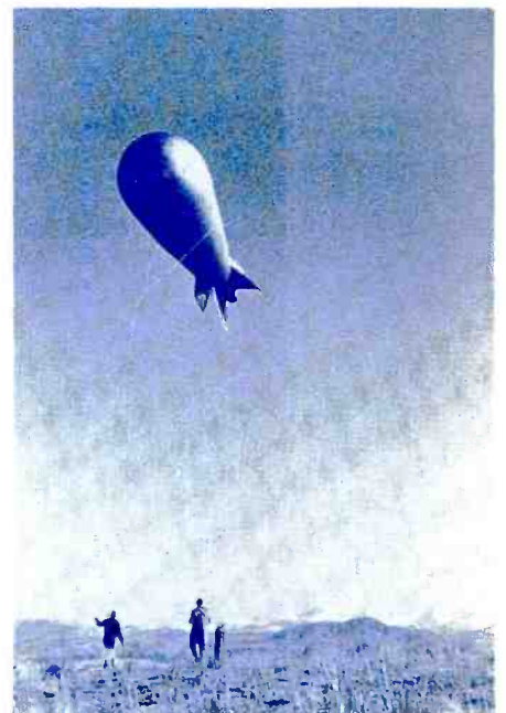
E. FLYING KITE SUPPORTING ANTENNA WIRE.
