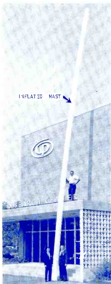
B. INFLATED ANTENNA MAST.
