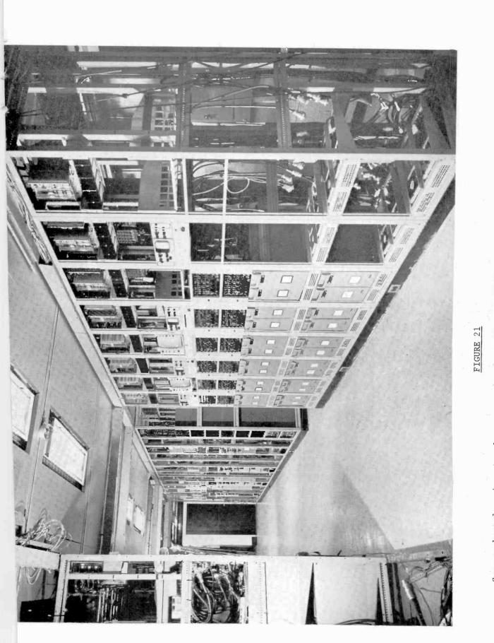
Camera channel equipment and pre-operational adjustment controls are centralized in the Equipment Center. Live camera controls are in the near group of racks; monochrome and color film channels in the farther group.
