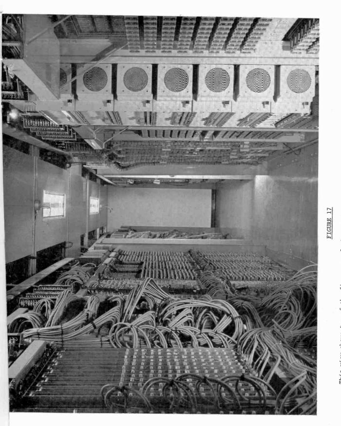
This view shows two of the five rows of wire-spring relay selector equipment which makes up the signal selection portion of the Master Exchange switching system. A total of 35,000 wire-spring relays are used to handle audio, video, and communications circuits.
